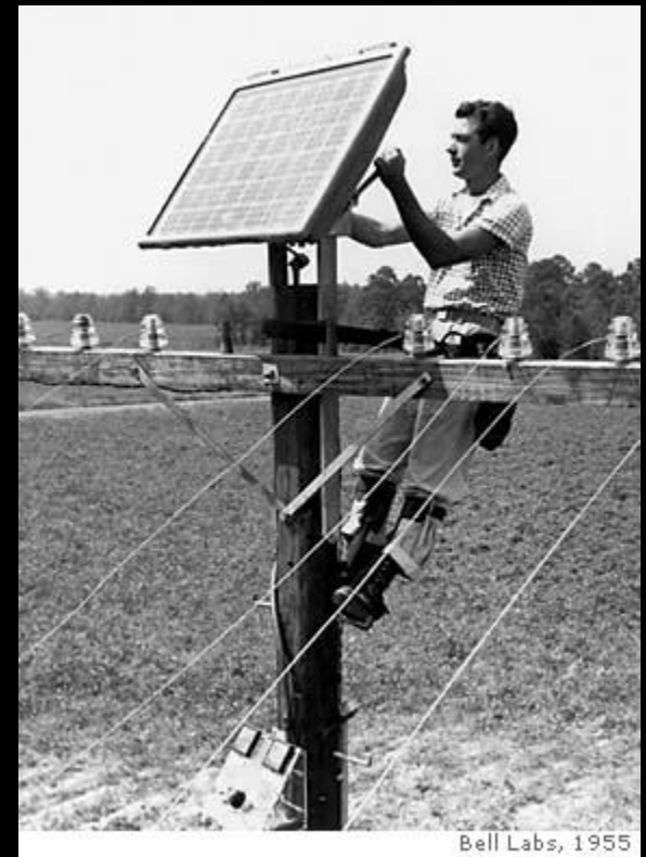
The original Bell Solar Battery (photovoltaic panel) is used in an early test in 1945
