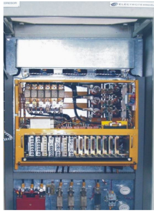
Fig. 12 The controlled rectifier as nonlinear load
