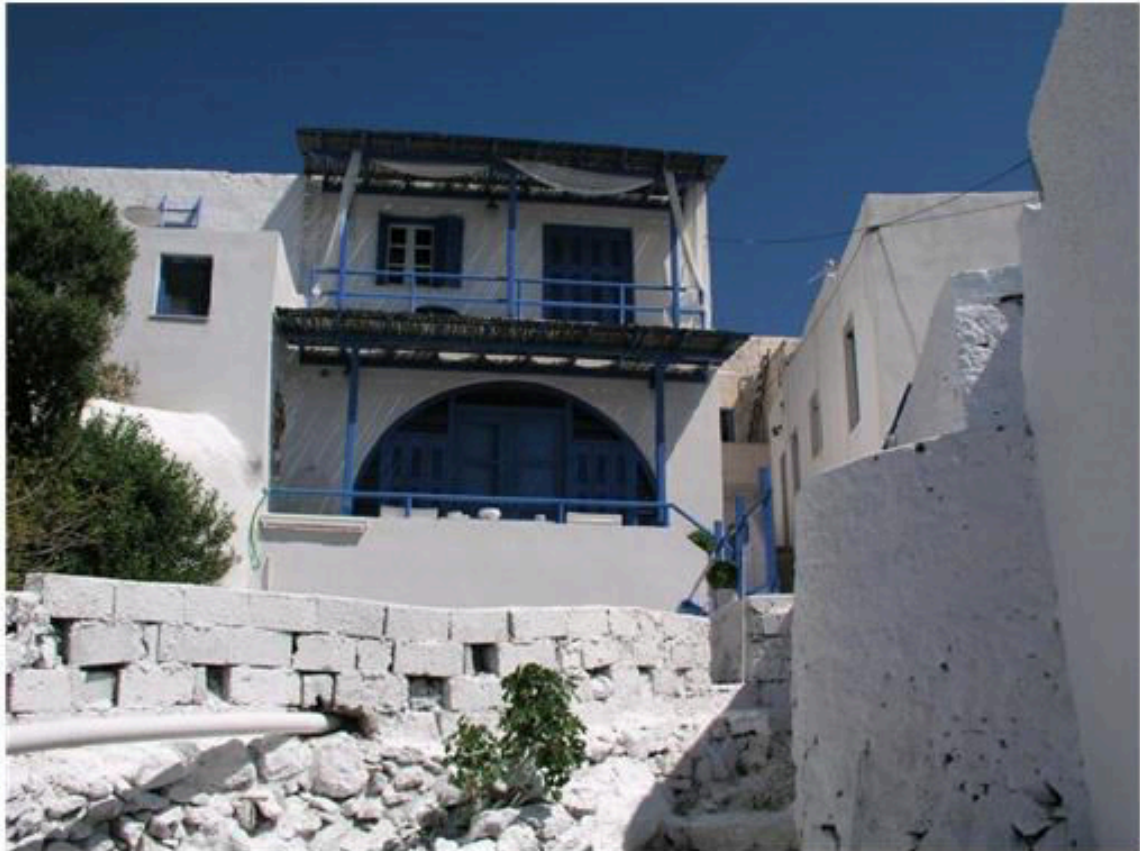
Island of Milos. A modern house adopting traditional forms (due to legislation imposing it). Vaulted loggia and cane shelter.
