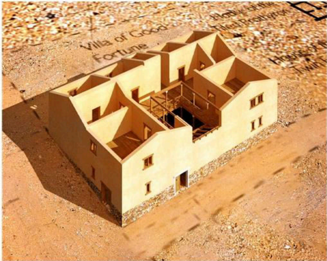
Villa of Good Fortune in ancient Olynthos. The walls of the first floor were entirely made of raw earth. The columns supporting the portico surrounding the court and its roof were made of wood.
