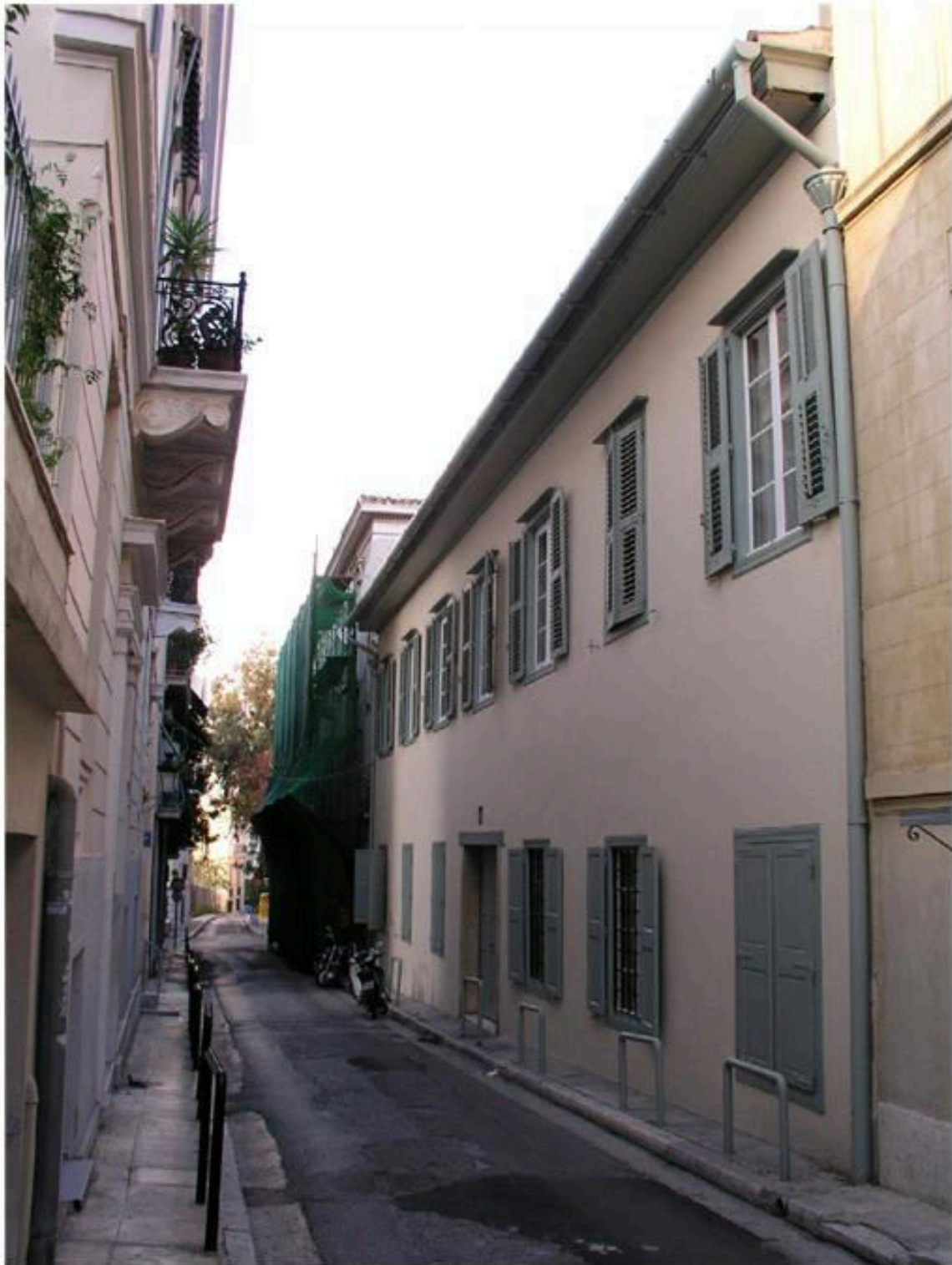
Athens. An example of a house hiding completely its traditional and highly bioclimatic layout behind its symmetrical and rigid façade. It is the house with the balcony closed with glass panes presented previously.
