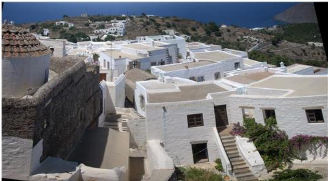
Islands of Santorini (above) and Patmos (below). The roofs have insulation made of earth and seaweeds and they are flat, in order to collect the rain water.
