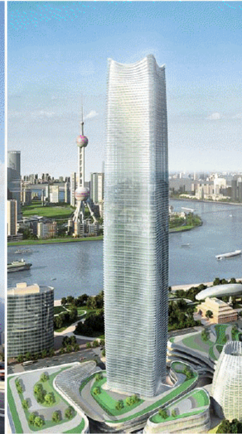
The North Bund White Magnolia Plaza Shanghai, China 320 m
